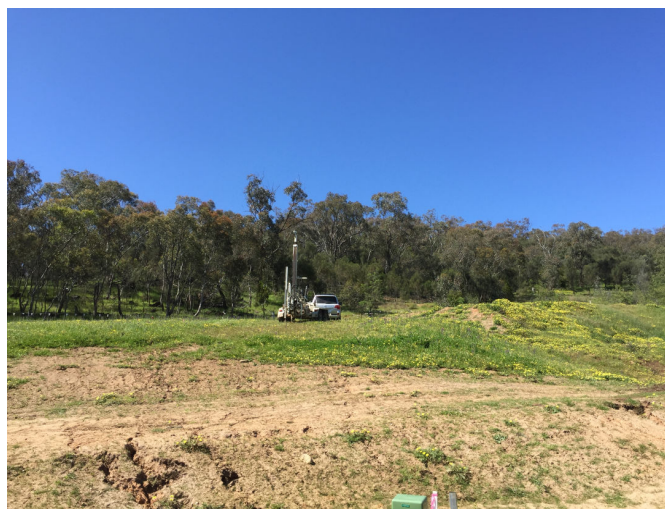
Existing site conditions for proposed dwelling.
